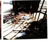
There are several pipe lines on this part of the bridge also kept exposed crossing through Footpath on this part of the bridge. The pipes arejust thrown without any proper management.
