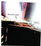
The cantilevers are fixed into the ground and right at the ground surface level some rust has started appearing needs to take care.
